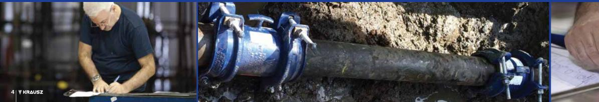
Patented sealing solution is the pressure-assisted gasket featuring two-stage sealing: mechanical sealing that is effective under vacuum or non-pressure, and self-inflating gasket using water pressure.
